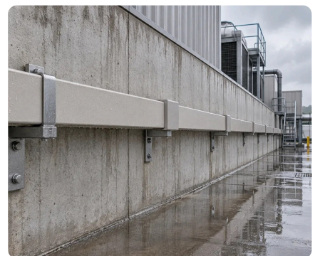
Outdoor and tunnels
