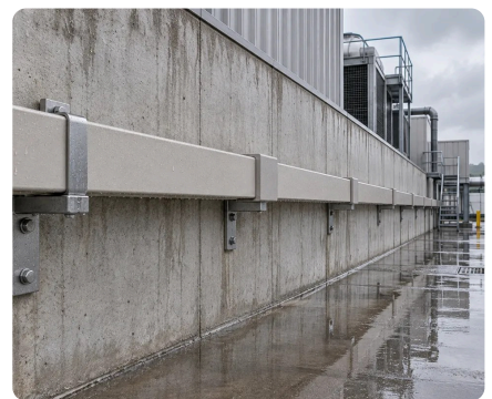
Outdoor and tunnels
